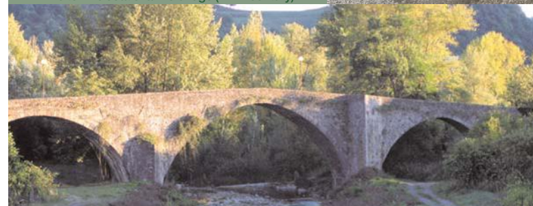
The town's coat of arms bridge (XIIIth century)
